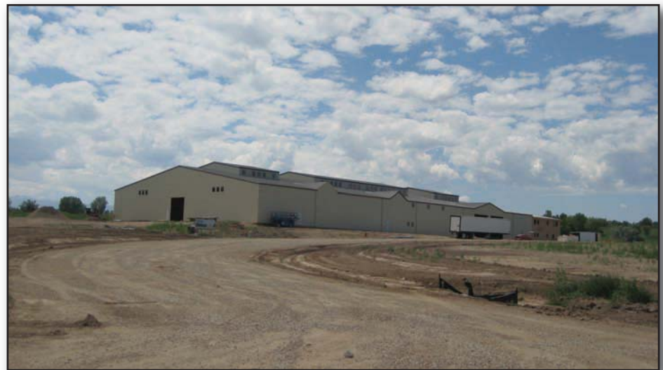
Vacu Tech building under construction
